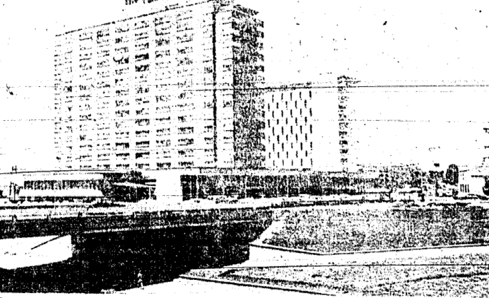
TYPICAL OF HOTELS awaiting tourists who travel through the big cities of South America is the Tequendama Hotel, pictured above, located in Bogota, Colombia. Food, service, shops and furnishings are, in essence, the same as in the same quality hotels in the United States . . . even to one-day laundry service.
