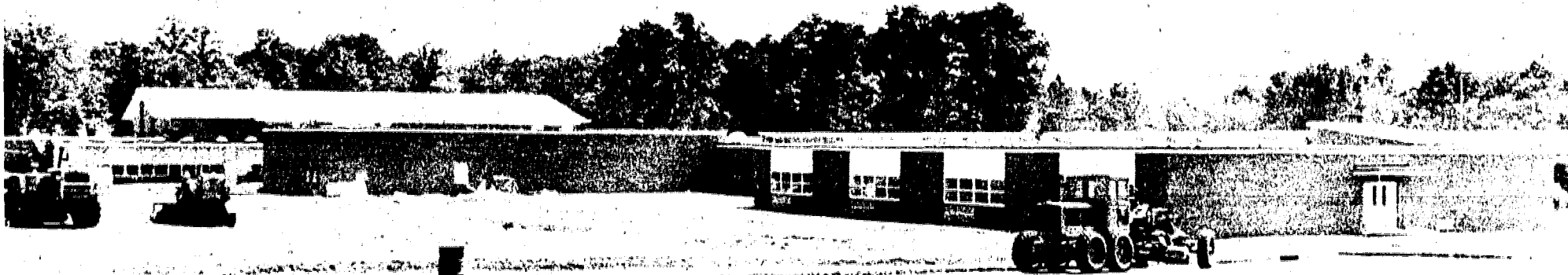
THE WORK GOES ON---Classrooms may be silent at Deerfield School, but the ground work goes on as crewmen seek to finish the almost completed work of paving. By September
