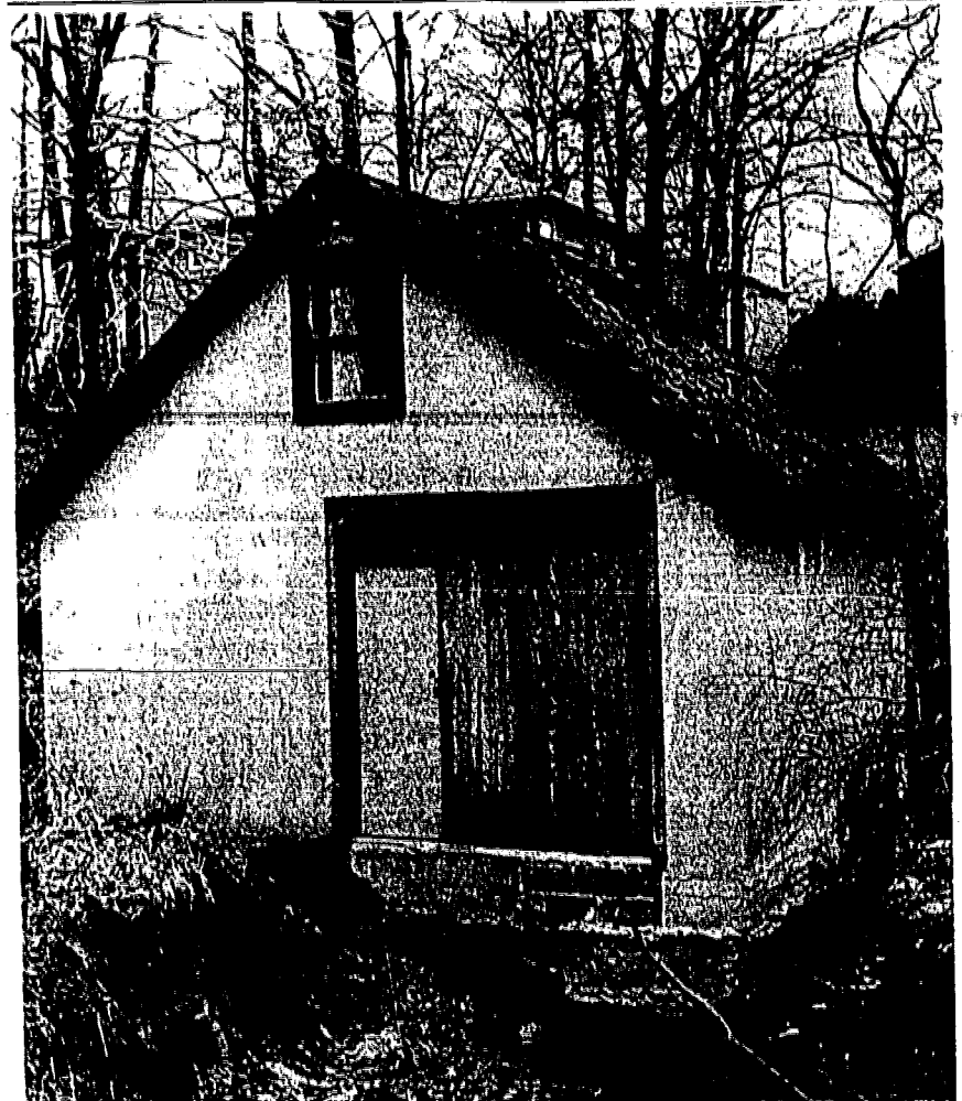
PERILOUS ROOF — An accident several weeks ago, in which a local eight-year-old boy was injured when he fell through the roof of this building, has spurred an investigation of other such buildings in the borough which might be hazardous. Results should be made public at the Borough Council meeting this Tuesday night.
