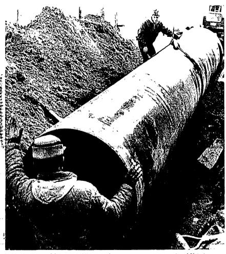
MORE PIPELINES FOR MORE WATER --- Construction crews put a section of 36 inch water main in place in Mountainside as work progresses on Elizabethtown Water's new six-mile pipeline from Scotch Plains to Kenilworth. The transmission main will bring additional water to Hillside and Union and strengthen supplies to Westfield, Mountainside, Kenilworth
