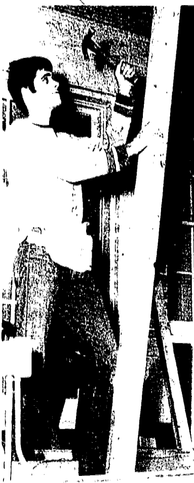
WORK STARTS on addition at Children's Specialized Hospital, New Providence road, Westfield. The specialized rehabilitation facility is expanding its present quarters in an effort to meet increased demands. The hospital now has a waiting list for patients.
