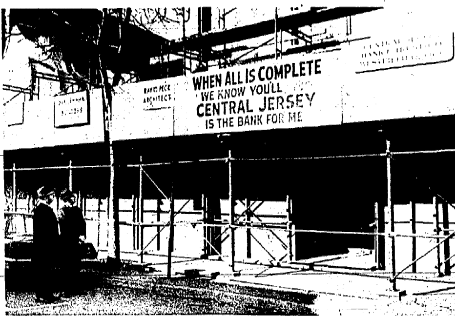
BANK REMODELS — Inspecting remodeling and renovation of the Westfield office, the Central Jersey Bank and Trust Company, are manager and executive vice-president Harry A. Giuditta, left, and vice-president Richard S. Pinnell. The bank is open to serve the public uninterrupted during the construction work, which is scheduled for completion within the next few months.
