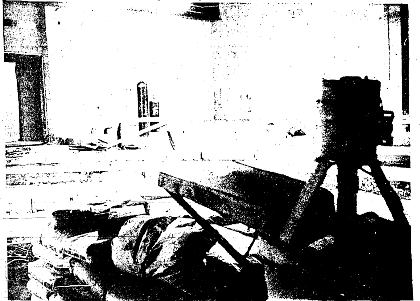
CONSTRUCTION SONG—The sound of construction equipment is echoing off the walls of the new music complex at Jonathan Dayton Regional High School these days. The complex, when completed, will house facilities for instrumental and vocal music instruction for students at the Springfield school.
