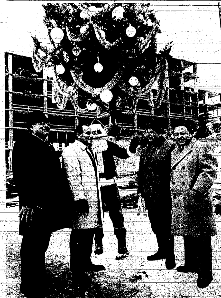
TOPPING OFF — Architect Thomas W. Moule of Mountainside, second from right, takes part in traditional topping-off ceremony at the Kim Institute of Rehabilitation Medicine, the 162-bed hospital being built by Motor Club of America on Central Avenue, East Orange. Moule, of T.W. Moule and C.W. Hoff, also designed the award-winning MCA national headquarters in Newark. Pictured from left: Bernard Burstein, MCA vice-president in charge of construction; Ben Torcivia, president of Torcon, Inc., general contractor; Santa Claus; Moule and Dr. Ki Ho Kim, medical director of the hospital.
