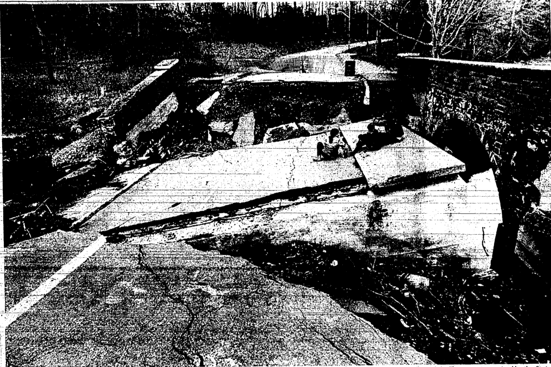
BRIDGE IN TROUBLE—A group of teenagers uses one of the washed-out bridges in Echo Lake Park as a gathering spot; it offers some measure of privacy since the road is still closed to vehicles, and other pedestrians are not likely to climb over the debris. A check last week with the Union County Park Commission on the progress of repairs to the two bridges, dam and retaining wall damaged in the Aug. 2 storm revealed that engineers are still in the process of drawing up plans for reconstruction. A commission spokesman said the designs are required by the State Water Policy Commission, which must approve them. Following that, bids must be advertised and cost estimates filed for approval with the Federal Disaster Agency, which would fund the work. The spokesman, noting he hoped repair work would begin by this summer, stated, "We are moving as fast as possible because we are interested in getting the park back to normal use." (Photo-Graphics)
