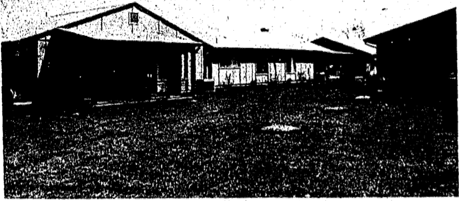
NOW AVAILABLE—Segment of Clearbrook, the 3,200-home adult condominium which Aaron Cross Construction Co. is developing off exit 8A of the New Jersey Turnpike in Monroe Township. Sales are now under way in the fifth section where homes are priced from $25,990 to $34,990 for adults 48 years of age and older.
