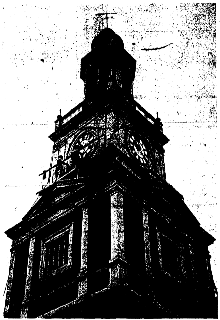
FALL COAT—A new paint job is applied to the Jonathon Dayton Regional High School in preparation for yesterday's school opening.
