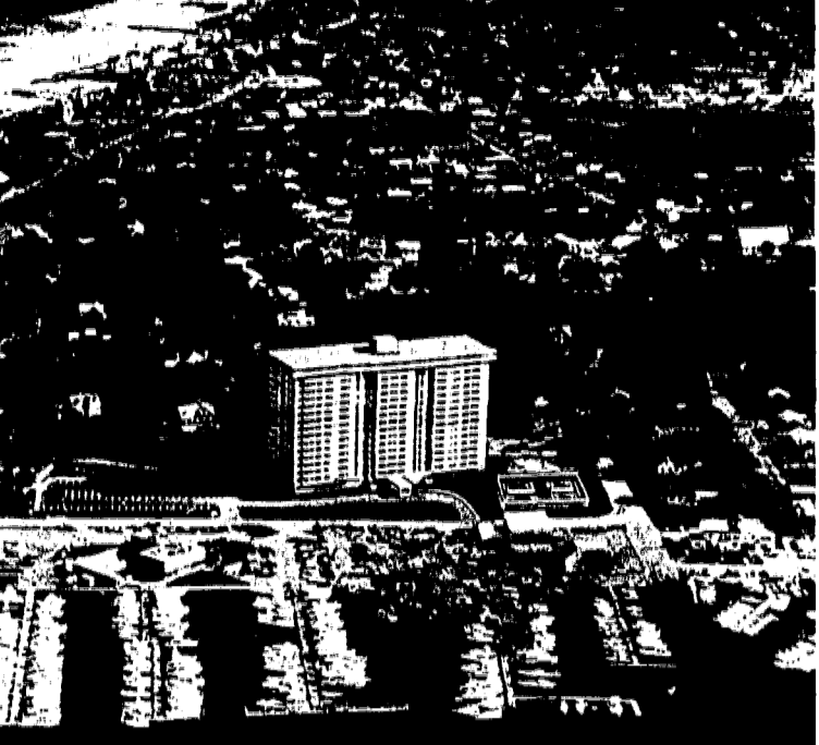
READY FOR SHOWING - The 17-story Channel Club Tower luxury condominium at Monmouth Beach is expected to be fully completed by the end of the year. Preview showings begin this month.
