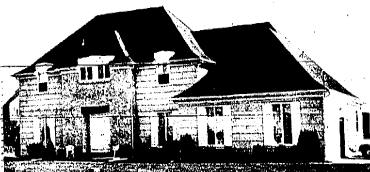
THE CHATEAU — This five-bedroom home is among five models offered at Palmer Hill Estates, a sub-division of 34 custom-built homes in West Long Branch. In addition, the developers have other plans available, or will build to suit the buyer's plans. Model homes range in price from $79,000 to $150,000.
