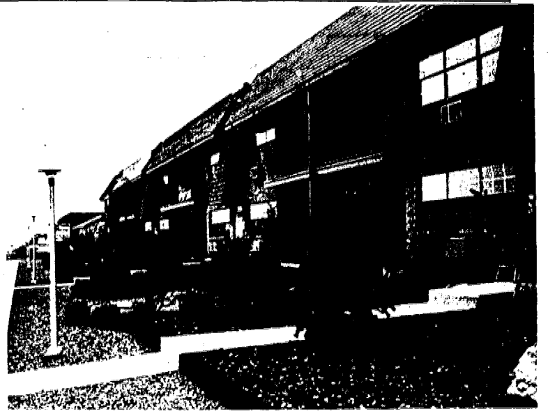
CONTEMPORARY STYLE — The Fountains, a new luxury condominium community on Ocean Avenue, Seabright, boasts the latest architectural look. Residents enjoy air conditioning, color coordinated kitchen appliances, future dock facilities, on-site swimming pool and private beach.
