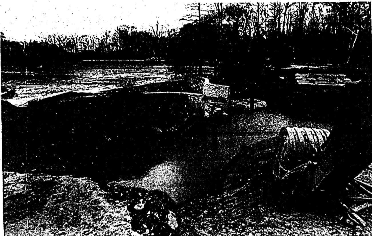
AT LONG LAST—Crane and pile drivers have been moved into Echo Lake Park for start of a $973,000 project to repair bridges and dams damaged in the Aug. 2, 1973, rainstorm.
