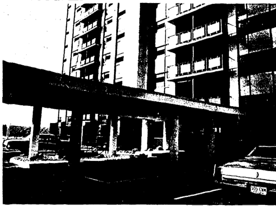
EASTPOINTE ENTRANCE — A covered walkway leads to the Eastpointe condominium building in Highlands, featuring 24-hour doorman service; heated Olympic-size swimming pool; security system; exercise and game room; saunas; appliance-equipped kitchens; oversize balconies; tennis courts; and laundry space in all apartments. The structure is owned by the General Electric Credit Corp., a subsidiary of the General Electric Co.
