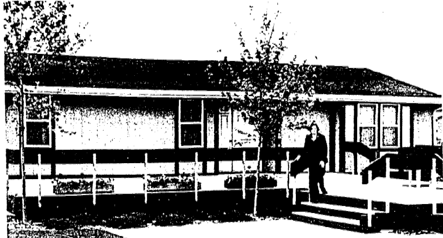
CLEARWATER GREENERY —Extensive landscaping work is in progress at newly-opened Clearwater Village, an adult mobile home community in Spotswood, which has eight model homes on display. Some homes in the nearly-completed first section of the development are ready for immediate occupancy.
