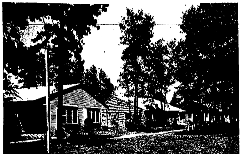
NEW MODELS—The Westbury model is in the foreground of this view of the new model area at Crestwood Village. It's a two-bedroom home featuring a colonial exterior and a one-story ranch layout. Other homes are throughout the rolling park-like area. 10 new models are open at the retirement community on Rt. 530 Whiting, all during the week from 9 a.m. to sundown.
