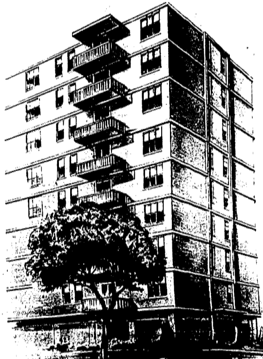
ELIZABETH CONDO —Polonaise II, a former rental building on N. Broad street, has been converted into a condominium, with two-bedroom apartment prices starting at $29,900. Six floor plans are available.
