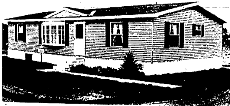
COLONIAL VILLAGE — Fully-furnished, insulated and equipped with the latest energy-saving systems, the manufactured homes of Colonial Village in Mt. Bethel, Pa., are priced from $22,364. Set on individual lots within an 82-acre private residential-recreational community just across the Delaware from New Jersey, the exceptionally-affordable homes are virtually indistinguishable from conventional Colonial ranch-style housing. After purchase of a Colonial Village home, residents pay lot charges of from only $119 per month for all community services, including security, recreational facilities, real estate taxes, sewers, water and street snow removal.
