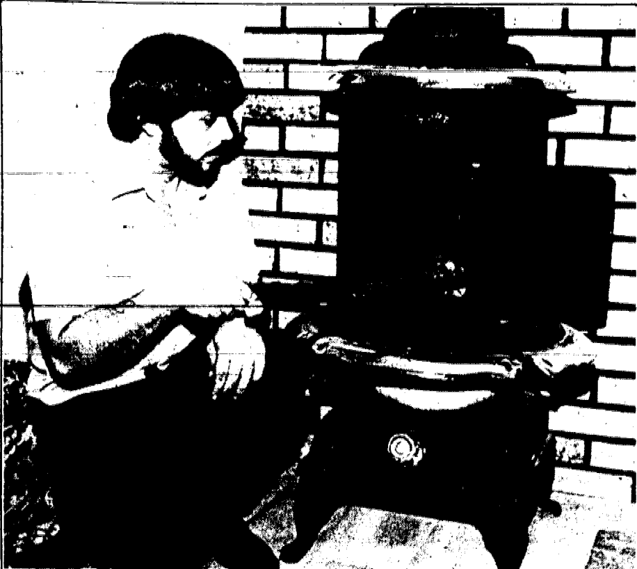
KEEPING WARM WITH WOOD — Doug Vetting of Roselle stirs the ashes in his pot-bellied stove. Vetting got a permit to burn wood in the vintage heater from his local building inspector, Frank Belluscio. He also went beyond the required safety specifications, installing a brick fireproof wall before putting in his stove. (Photo by Roy Graves)
