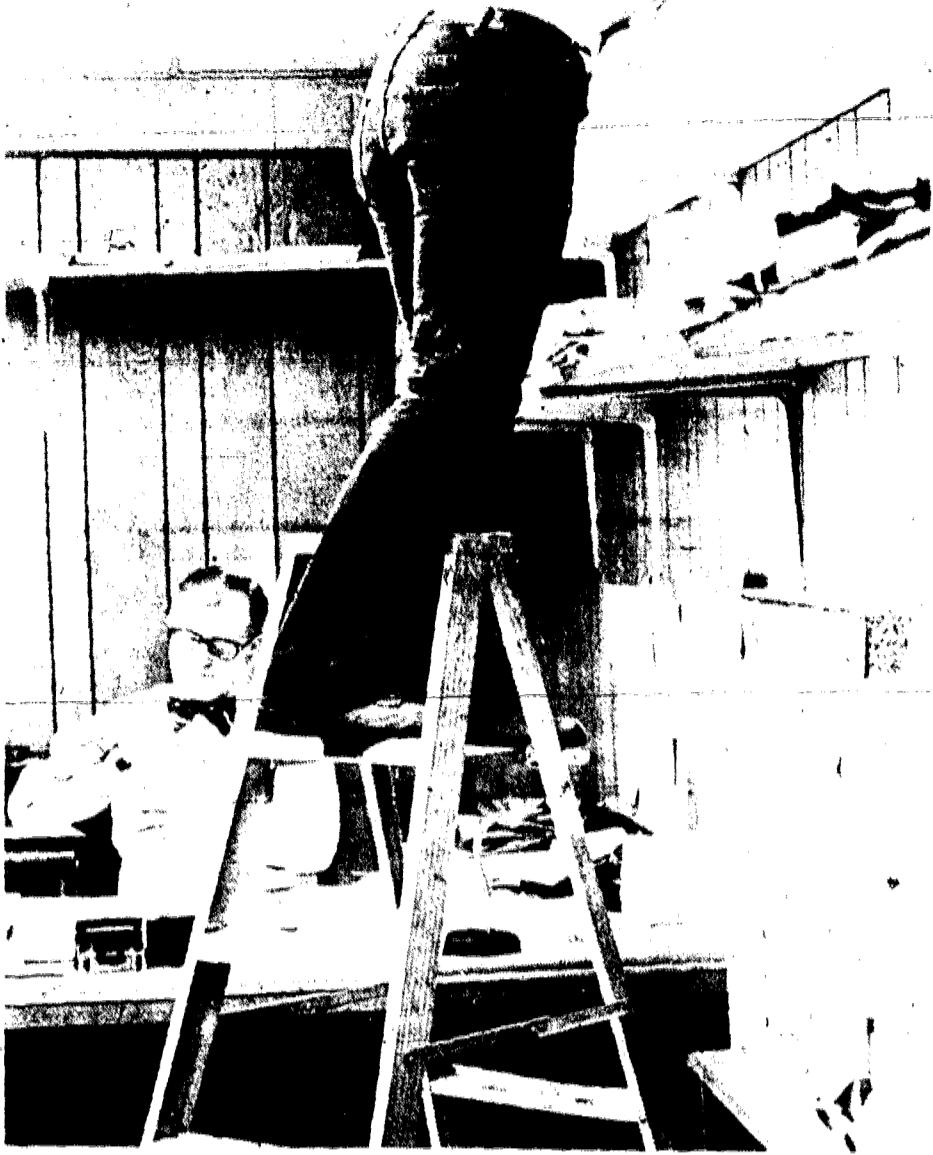
GETTING TO THE TOP —Stan Gibson, installer for Mycro-Tek Inc., runs wiring through the ceiling while Bob Brumell, vice president of advertising, works in the background.
