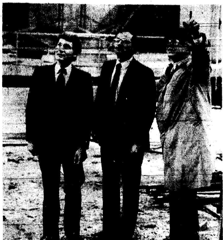
SENATOR RECEIVES UPDATE ON PLAYHOUSE RECONSTRUCTION —Senator Donald Di Francesco (R-22), center, takes a tour of the construction site of the Paper Mill Playhouse, Millburn, scheduled to reopen in November 1982. With him are Angelo Del Rossi, left, executive producer, and Floyd H. Bragg, chairman of the board of trustees.
