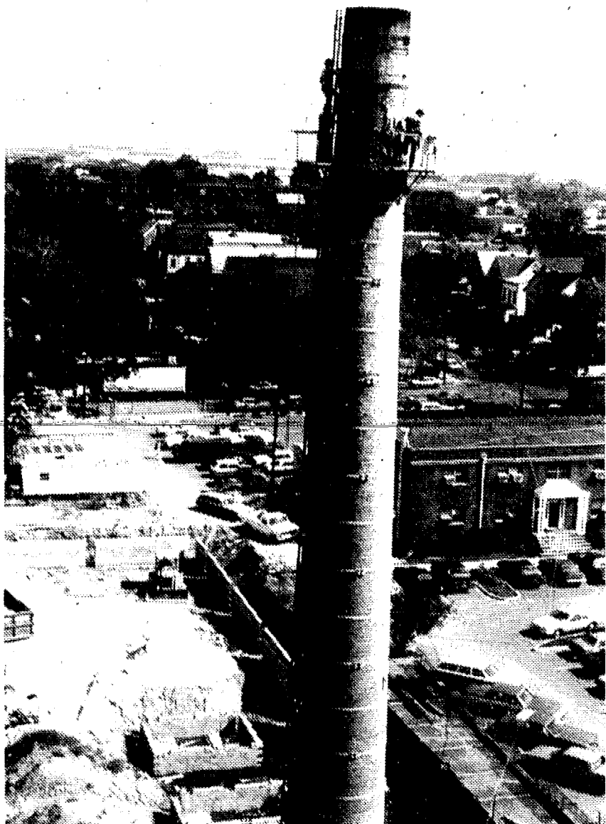
BIRD'S EYE VIEW —of Elizabeth General Medical Center's construction/renovation project is enjoyed by workers putting the finishing touches on the restoration of the medical center's seven-story smokestack. A new intensive and coronary care unit, short-stay unit and adult psychiatric unit are among improvements planned. The project will be completed in 1988.
