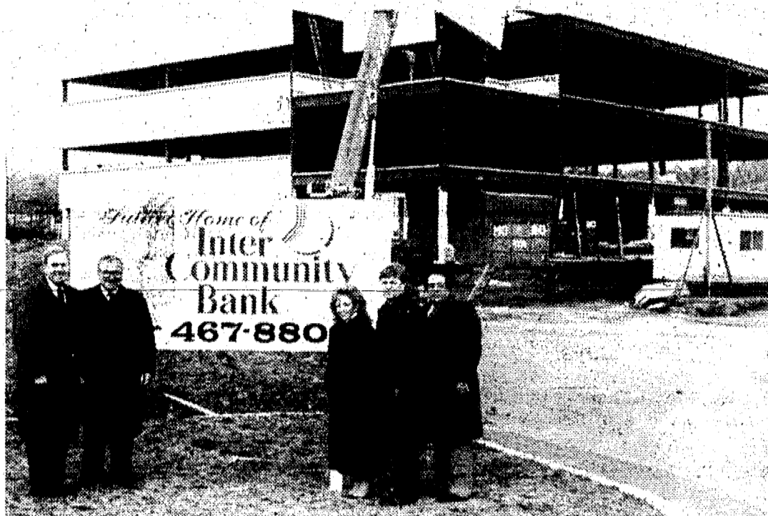
GOING UP — At the construction site of Inter Community Bank's new office in Springfield are, left to right, Jerome Waldor, bank chairman; Nazario Paragano, bancorp chairman; Denise Casale, branch manager; Mark Fogt, president and chief executive officer; and Michael Bono, senior vice president, sales and marketing.
