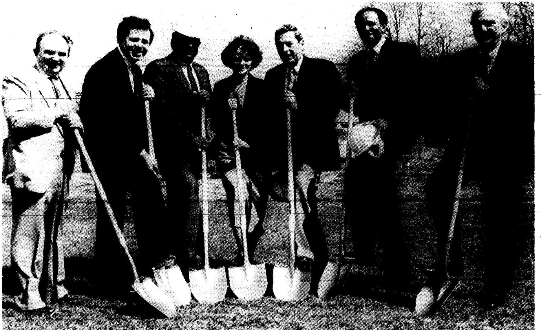
DIGGING IN — Jeanne Stamler, center, wife of county Prosecutor John Stamler, prepares to break ground for the new Union County Police Academy in Scotch Plains on Friday. Assisting are, from left, county Free-
