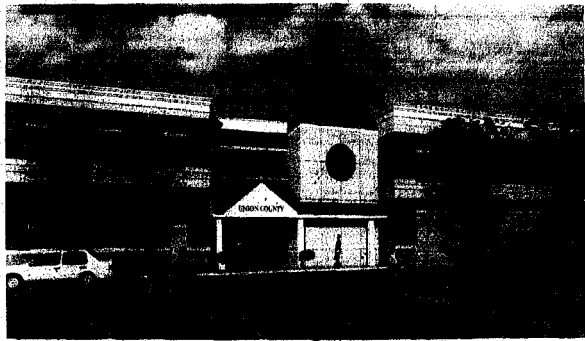
Renovations are planned for several county buildings, including the Venerri Complex in Westfield which houses the County Police. Construction is expected to begin on several projects in 2000, including a new juvenile detention facility and continuing renovations to the county courthouse.
