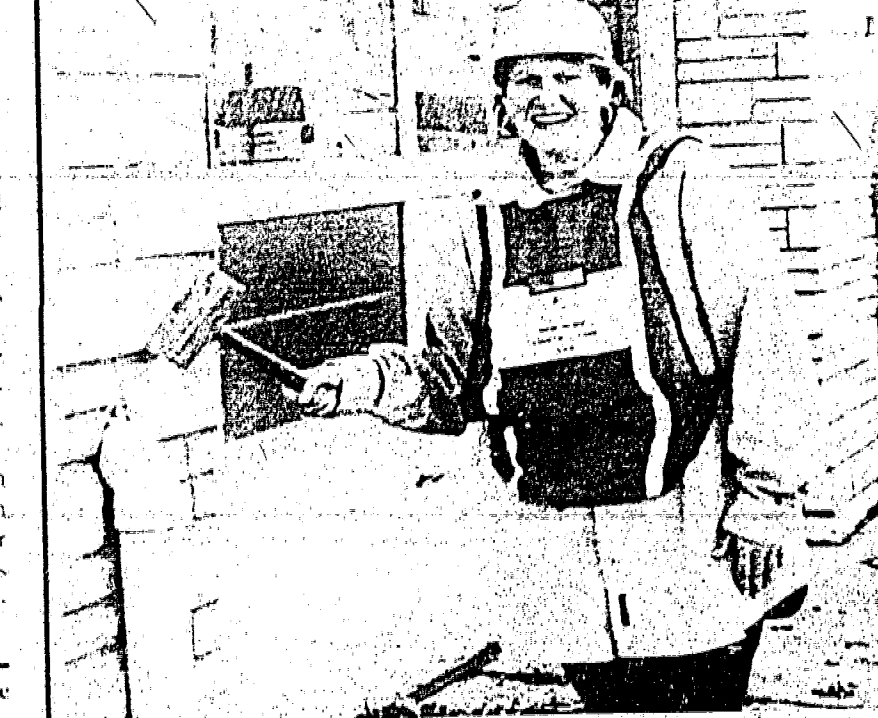
Kathy Lyons, director of SAGE Home Care, dons construction wear for Halloween and shows her willingness to participate in the demolition of the building at 290 Broad St., Summit, in preparation for the construction of SAGE's new headquarters on the site. Groundbreaking ceremonies for the new headquarters are scheduled for Dec. 3 on the site.
