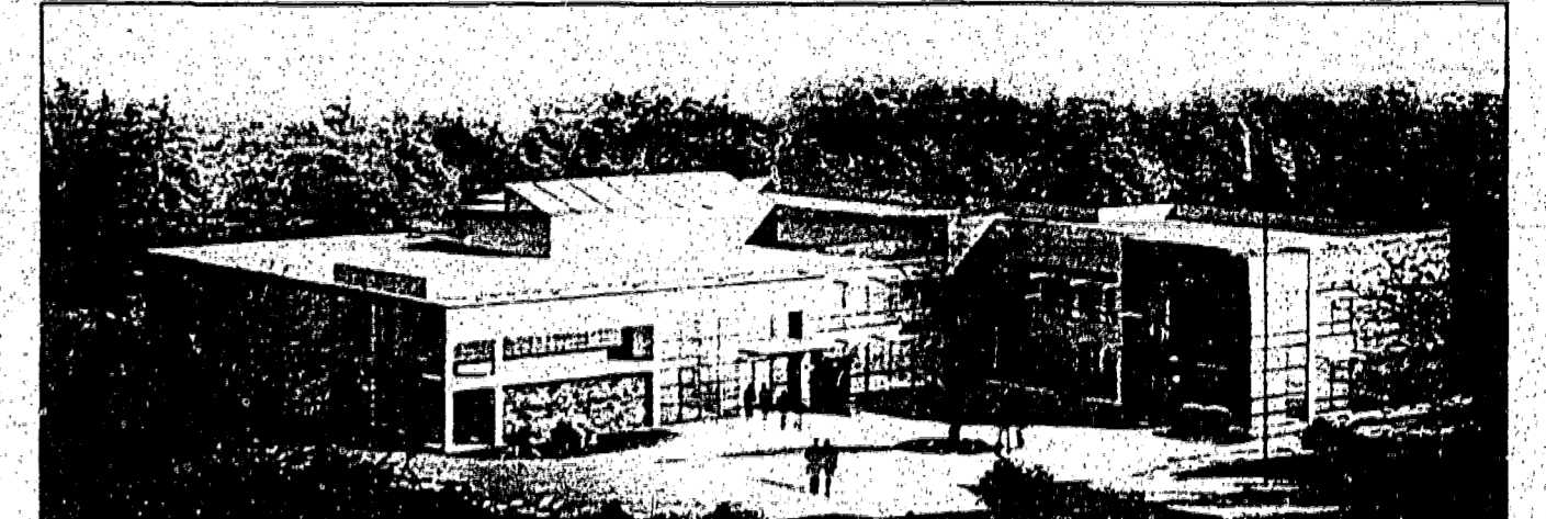
Union County's plans for Trailside Nature and Science Center in Mountainside will bring the facility to more than 25,000 square feet. Construction on the $5-million expansion is under way and expected to last 12 to 18 months.
