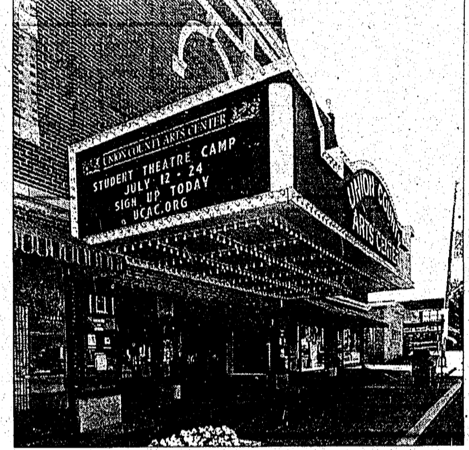
Although a study suggests approximately $16 million in various improvements to the Union County Arts Center in Rahway, county officials have only committed to the first phase, about $6 million, once it is acquired.
