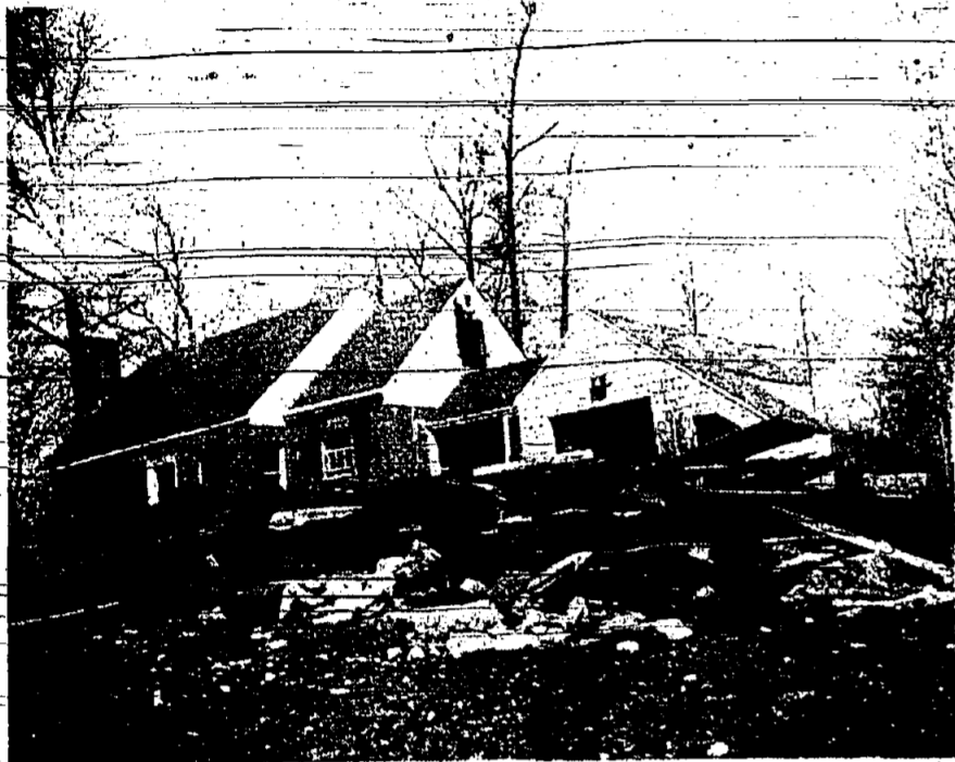
HERE WE GO AGAIN!—Litter covers the lawn of this state-owned house on W. Bryant ave. Windows are broken and the place is in a general state of disrepair. The Township Committee has, for the second time, requested that the State Highway Department take action in cleaning up property along the path of Rt. 78.
