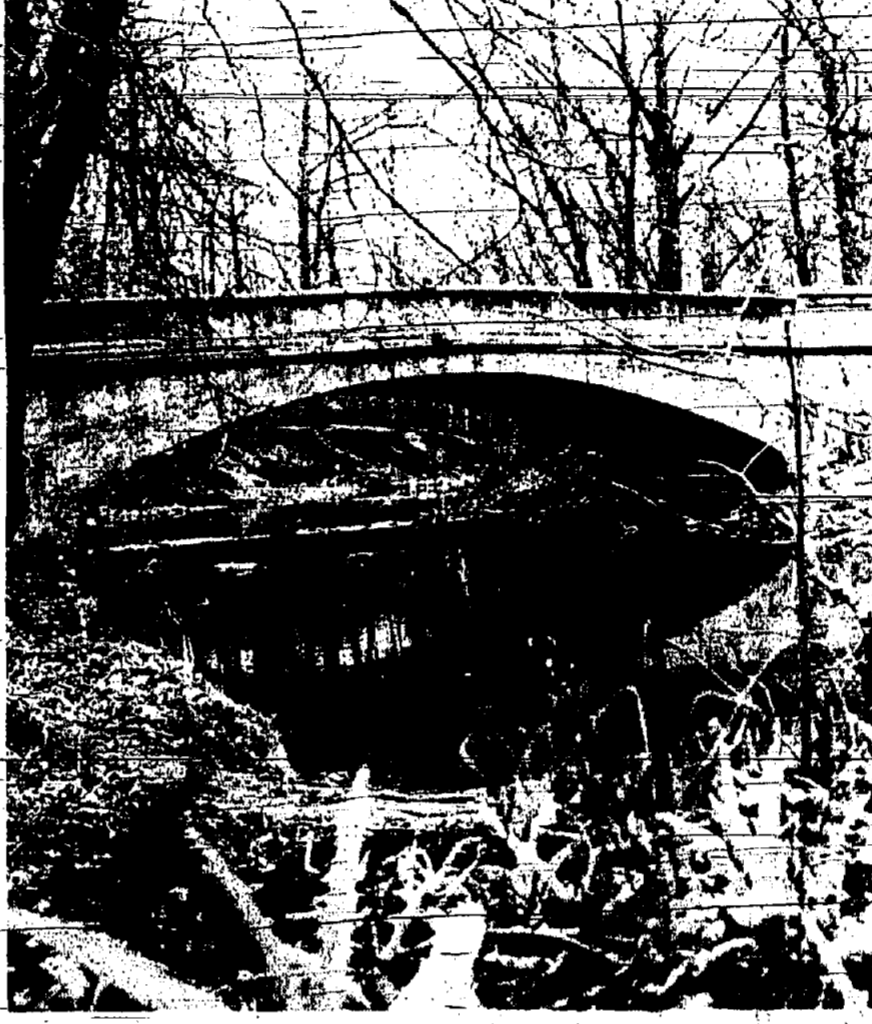
MILLTOWN RD. BRIDGE—The bridge spanning the Rahway River at the Springfield-Union line makes a picturesque scene, but not for long. The hazardous road conditions at the bridge will be eliminated—and so will the bridge. A newly aligned Milltown rd. and new bridge is in the planning stages, with completion slated by Dec. 1.
