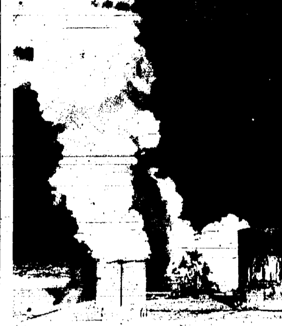
AT WAIRAKEI, in the center of the North Island, underground steam is tapped by deep bores and its great heat and pressure converted into electricity. Concrete cylinders of the type shown are used as silencers to deaden the tremendous noise of the escaping steam. (The noise, even so, still is impressive.)
