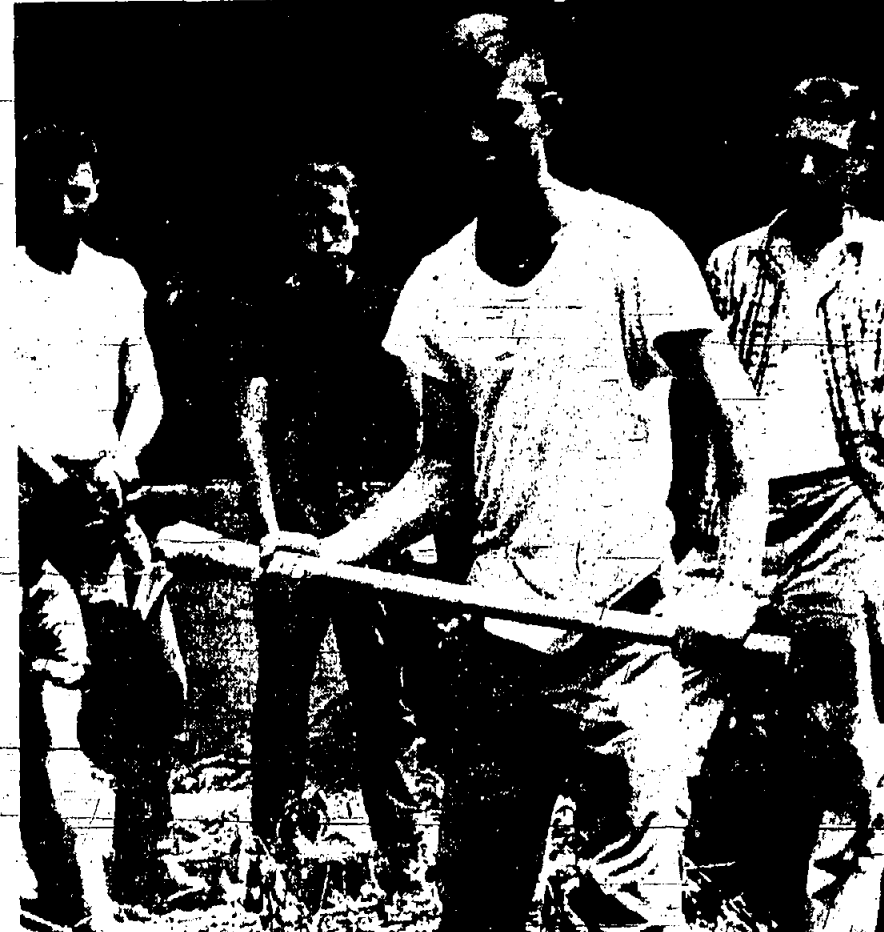
'OPERATION WORK' — John Guidara of 1233 Commerce ave., Union, in foreground, prepares to shove away debris along the Rahway River bed as part of the Union County Park Commission's five-week summer Youth Work program. This scene was taken at the Milltown dam, which straddles Union and Springfield. (Photo by A.H. Sicker)
