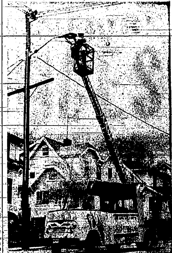
MODERN DAY STREETLIGHTER — Jersey Central Power and Light Company's new streetlighting replacement truck, which recently made its debut on Morris County streets, is shown as its operator changes one of the more than 17,000 streetlights in the county. The truck, according to utility officials, is designed to provide the safest and most efficient streetlighting maintenance.
