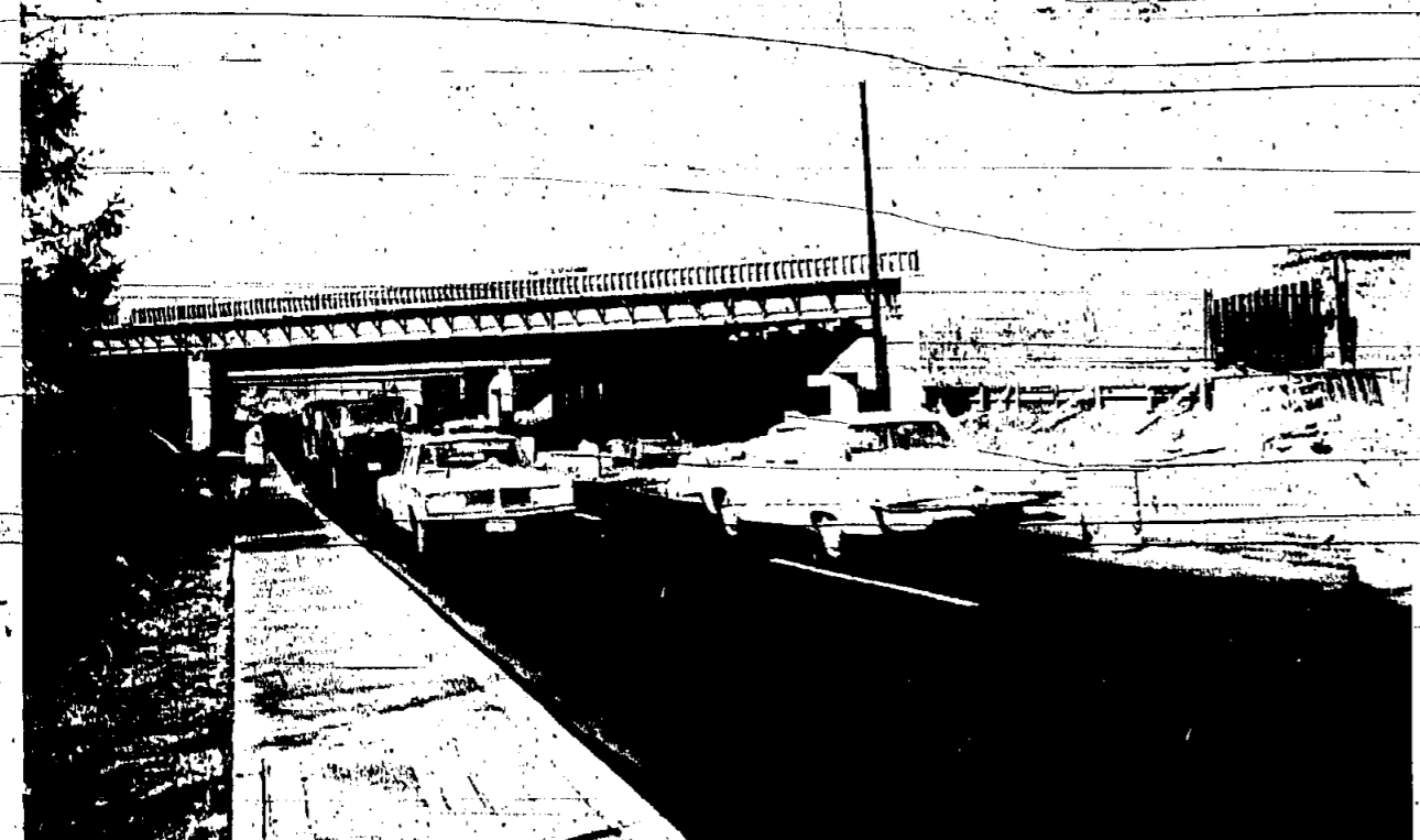
ROADBLOCK UNBLOCKED -- Morris ave. traffic last week flowed unhindered below the new bridge for Route 78, for the first time in approximately a year. The superhighway will be continued over the gap at right, where all cars driving along the main thoroughfare had been detoured on Morrison rd. The opening of the new segment of Morris ave. foreshadows the end of the emergency school bus service conducted by the Township Committee for the past year to transport youngsters across the hazards of the highway construction area. (Photo by Bob Baxter)
