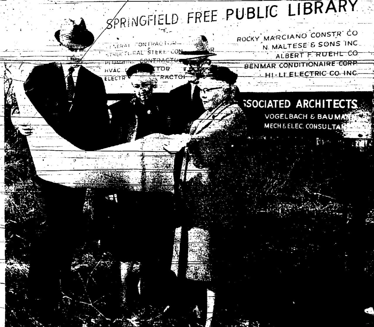
GROUND-BREAKING -- Looking over plans for the new Springfield Free Public Library, at ground-breaking exercises last Friday at the new library site at Mountain ave. and Hamphire st., are, from left, Robert Halsey, library board president, Phoebe Briggs, former township librarian; Don Palmer, curator of the library museum, and Mrs. A.B. Anderson, who headed the committee for Springfield's first library in 1932. (Photo by Bob Baxter)
