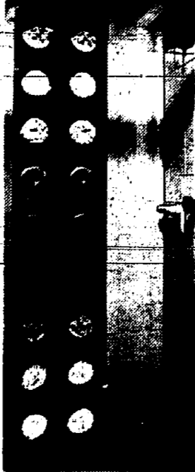
SHOWER STALL gets benefit of natural light, plus attractive appearance, with a vertical strip of glass blocks. In Intaglio pattern, from Pittsburgh Corning.
