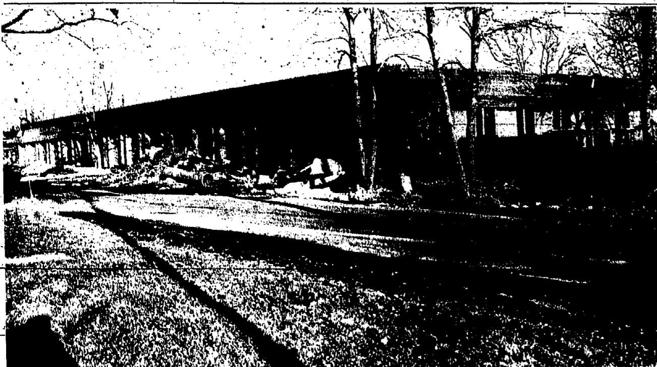
MAKING PROGRESS—With the exterior virtually completed for the new Springfield Library at Mountain Avenue and Hannah Street, work inside the building will be able to continue through the winter months. Completion date for the building is now tentatively set for April.
