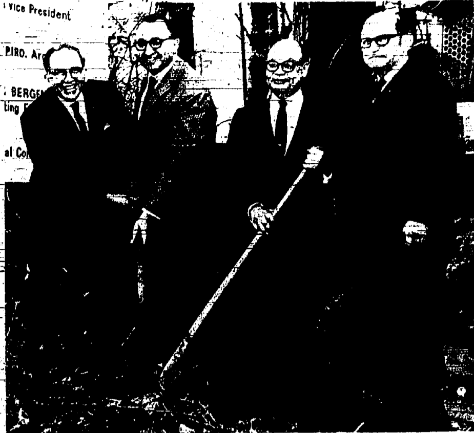
RUTGERS MILESTONE—Leaders in the drive for long-planned Rutgers-Douglass B'nai B'rith Hillside Foundation in New Brunswick are shown at construction site. Shown, from left, are Sidney Pillar of Springfield, Hillside chairman of Northern Jersey Council of B'nai B'rith; Phillip Lax of Maplewood, executive vice-president of the Building Corporation; Attorney General Arthur J. Silas, president of the corporation, and Morris Rohrbach of Newark, past president of the Northern Jersey B'nai B'rith. After 13 years of planning by more than 30,000 B'nai B'rith men and women in New Jersey, construction of the $1 million facility to serve 2,100 students at the state university is now under way. A September opening is expected.
