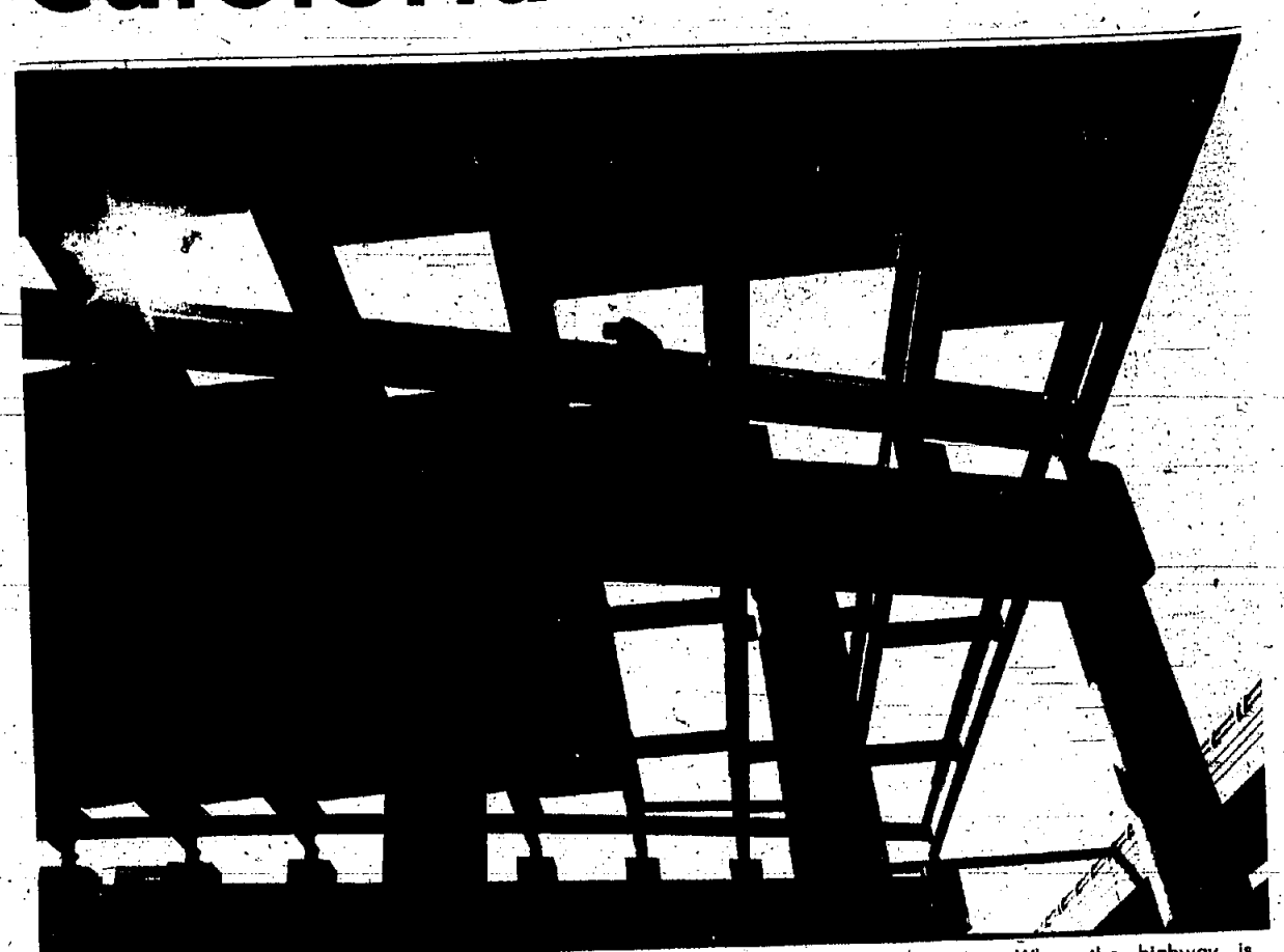
BRIDGE OVER STONEHILL ROAD is among Route 78 structures now being built in Springfield. The segment of the east-west freeway which cuts through the township is about 65 percent complete, according to officials of the State Department of Transportation. When the highway is finished, it will cross the state from the Holland Tunnel to the Pennsylvania line. It is open to traffic from Berkeley Heights west, but the section east of that point has been plagued by repeated delays.
