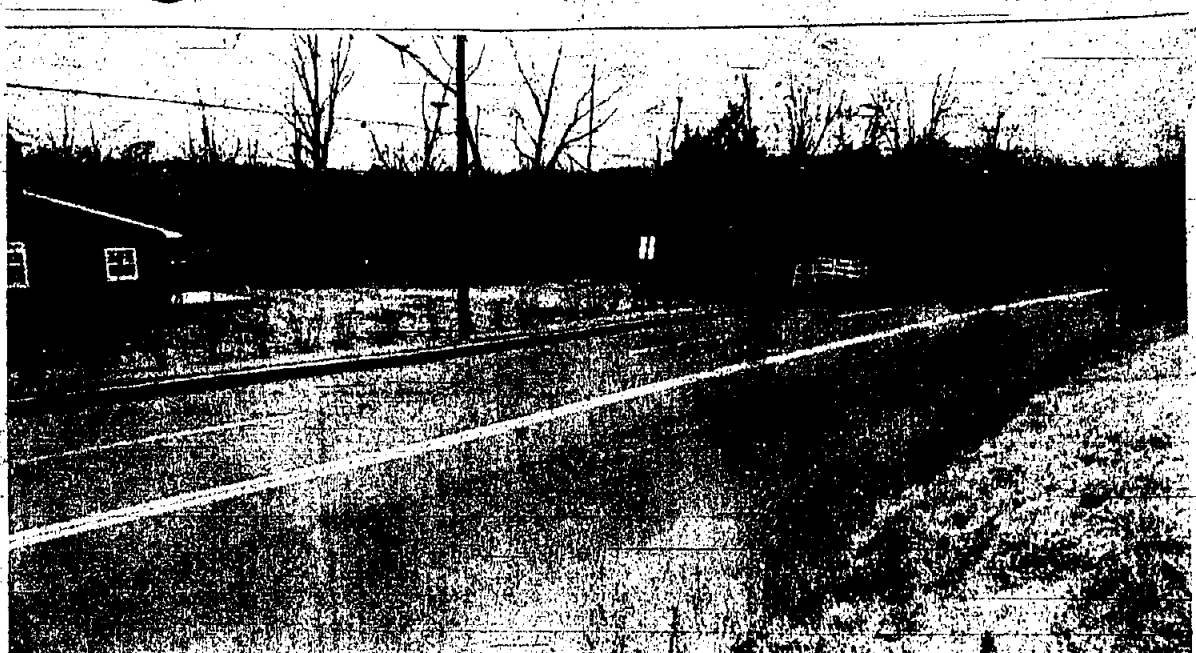
SCENE TO CHANGE — This view from Summit road just north of Little Brook road shows where Rt. 78 will leave Springfield heading toward the Watchung Reservoir. The environmental impact statement recently issued by the Department of Transportation stated that homes in this area will be affected by noise and some air pollution, as well as obstruction of the view. (Photo-Graphics)
