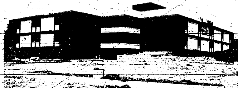
READY IN SEPTEMBER — Union County Technical Institute's new Allied Health Building, which will be ready for occupancy in September, will provide a dental clinic, open to the public, and house nine allied health programs.
