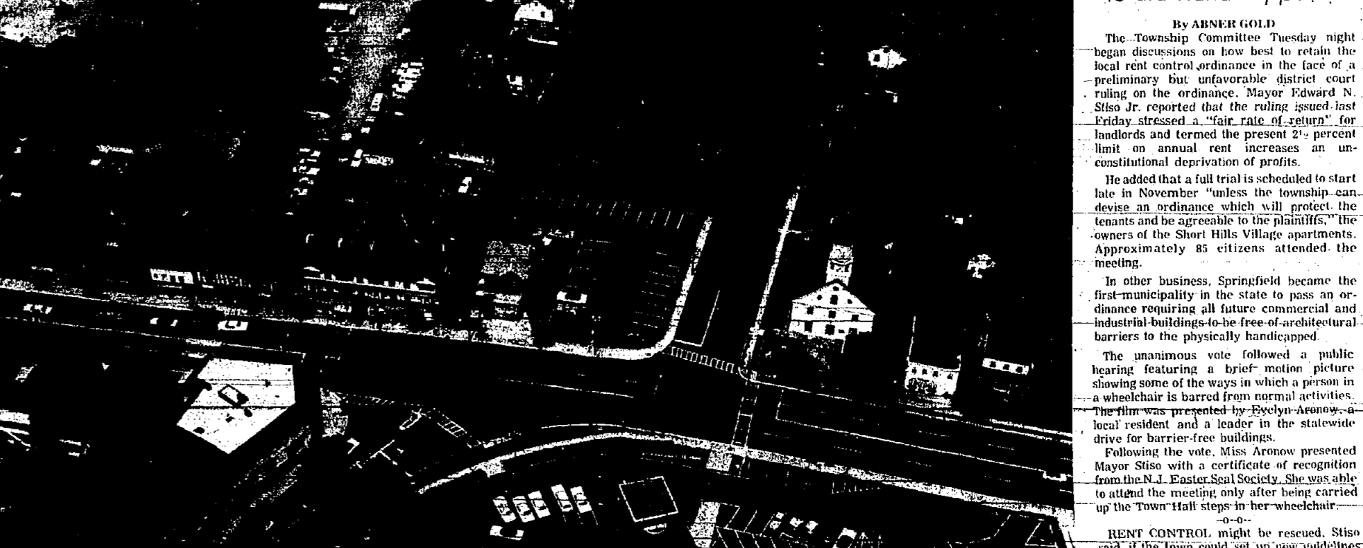
ROOM TO REDEVELOP — The Springfield Chamber of Commerce has urged the Township Committee to go ahead with plans now in the preliminary stage for the redevelopment of the Morris avenue business district. The plans call for demolition of most of the stores along the main thoroughfare and utilization of all the space extending back to Rt. 78, or rear. (Photo by Andrich Studios)
