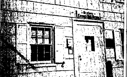
NEW SHUTTERS - The cannon Ball House has a new look, thanks to shutters installed recently on the landmark structure on Morris Avenue.
