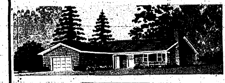
Featuring dramatic cathedral-ceiling living room with floor-to-ceiling brick fireplace.
