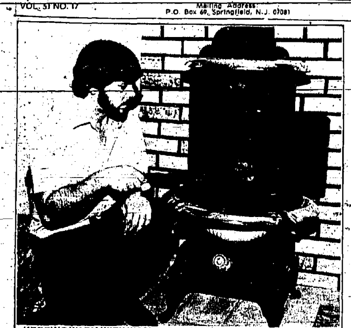
KEEPING WARM WITH WOOD - Doug Velling of Roselle stirs the ashes in his hot-boiler stove. Velling got a permit to burn wood in the vintage heater from his local building inspector, Frank Bellusco. Also want beyond the required safety specifications, installing brick fireplace before putting in his stove. (Photo by Roy Graves)
