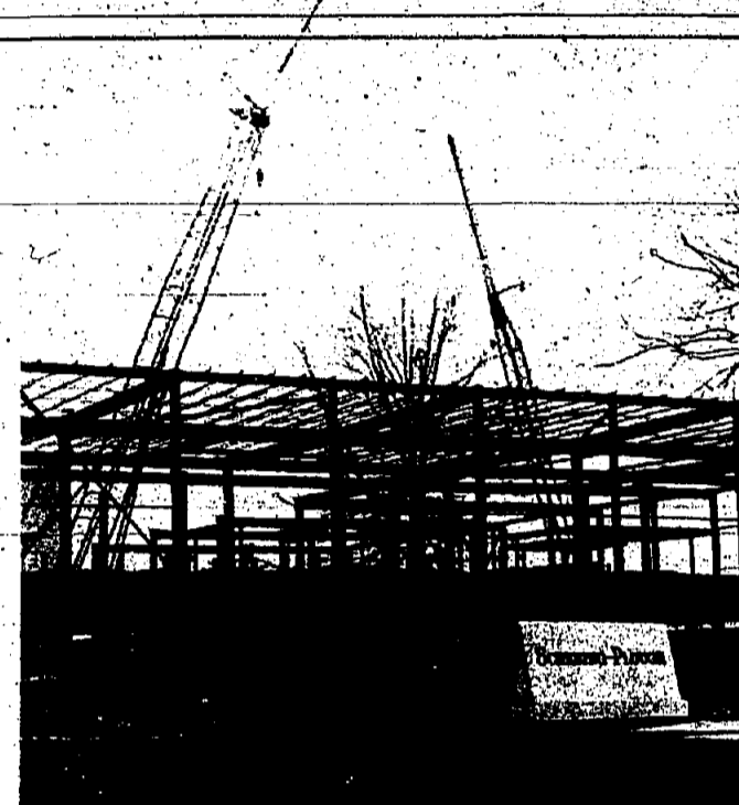
ADDITION UNDER CONSTRUCTION—Schering-Plough Corp. in Kenilworth is in the midst of building a multi-story addition.
