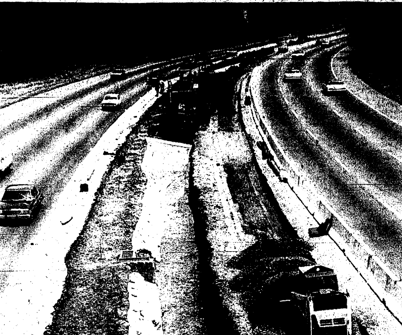
RUSH HOUR MADNESS which motorists now encounter on the Garden State Parkway in the Union-Essex counties area may be eased somewhat when construction is completed. This particular section, where bulldozers are leveling the ground in order to add a fourth lane to both the north and southbound sides of the highway, is in Irvington. It is coming along with 'no major problems' according to Adam Samiec, Irvington township engineer. Construction is expected to be completed sometime in 1985.
