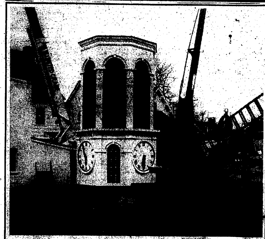
THE STEEPLE CHASE is on as workers prepared Friday to mount a new aluminum steeple, a replica of the former 200-year-old wood top, on the First Presbyterian Church on Morris Avenue and Church Mall. (Photo by John Boutsikaris)
