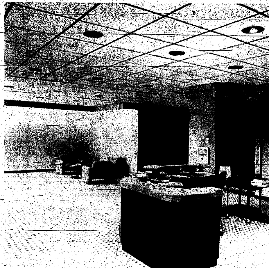
A VACANT WAREHOUSE ...is what Brown and Matthews transformed into modern office space for American Hoescht's ENCO Printing Division. The design/build firm brought the outdoors inside with an interior walkway, recessed lighting, live plants and colorful interior panels.
