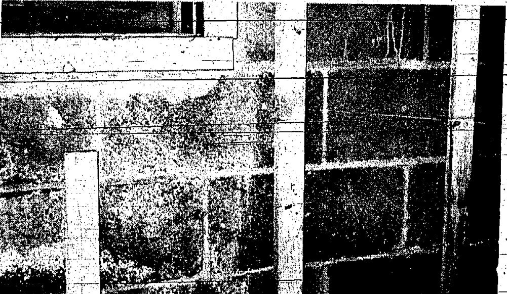
BARE WALLS —This is the view of one basement in the Pineview Garden complex on S. Springfield Avenue, which was found to be in violation of a township ordinance in regard to tenant service and building maintenance by the Rent Leveling Board. The panelling that once covered this cinderblock wall was removed at the request of a tenant, after mold from excess moisture began appearing.
