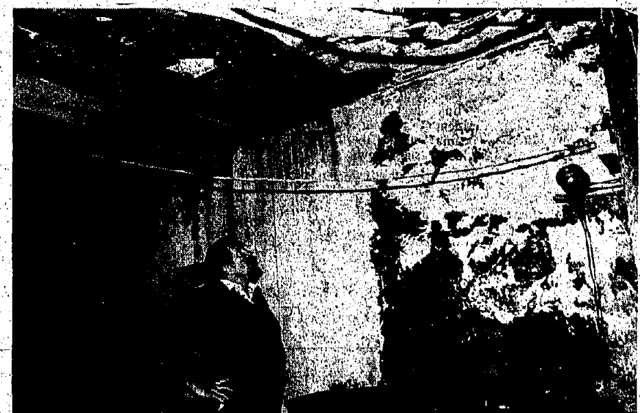
THERE'S WORK TO BE DONE—Dan Johnson, campaign director for the Union County Arts Center, inspects the alcove left of the stage which needs to be replastered and repainted.
