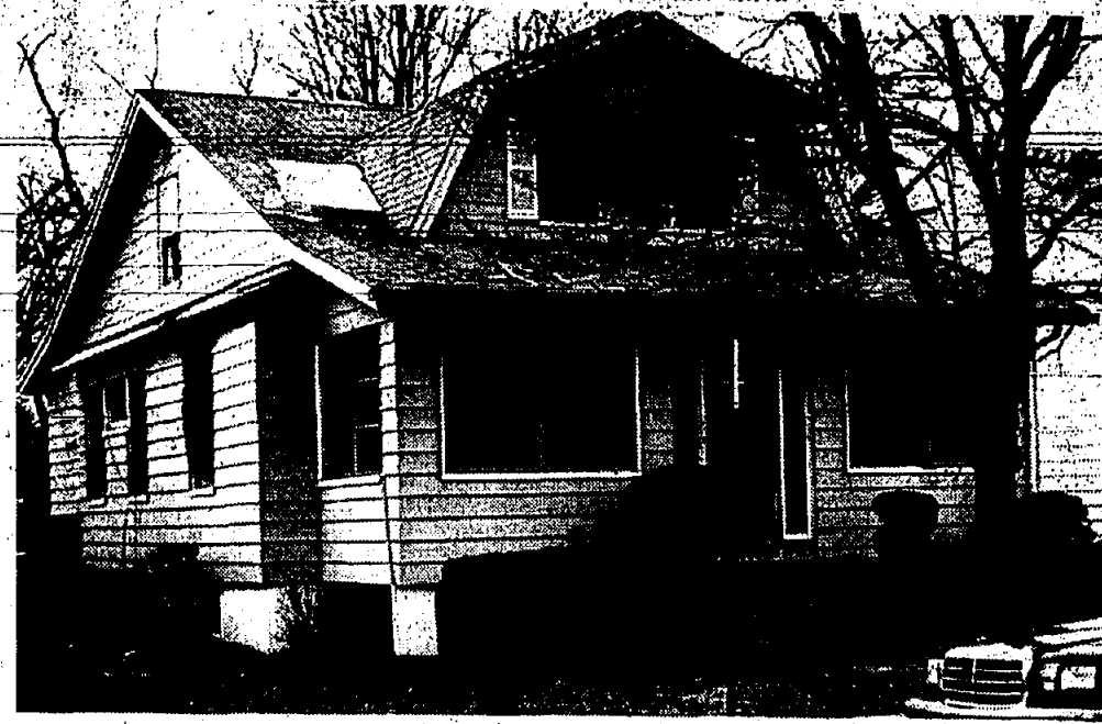
GUTTED HOME — This two-story frame home on Rose Avenue is where Josephine Slenkiewicz, a long-time Springfield resident, was overcome from smoke inhalation following a fire. She later died at Overlook Hospital in Summit.
